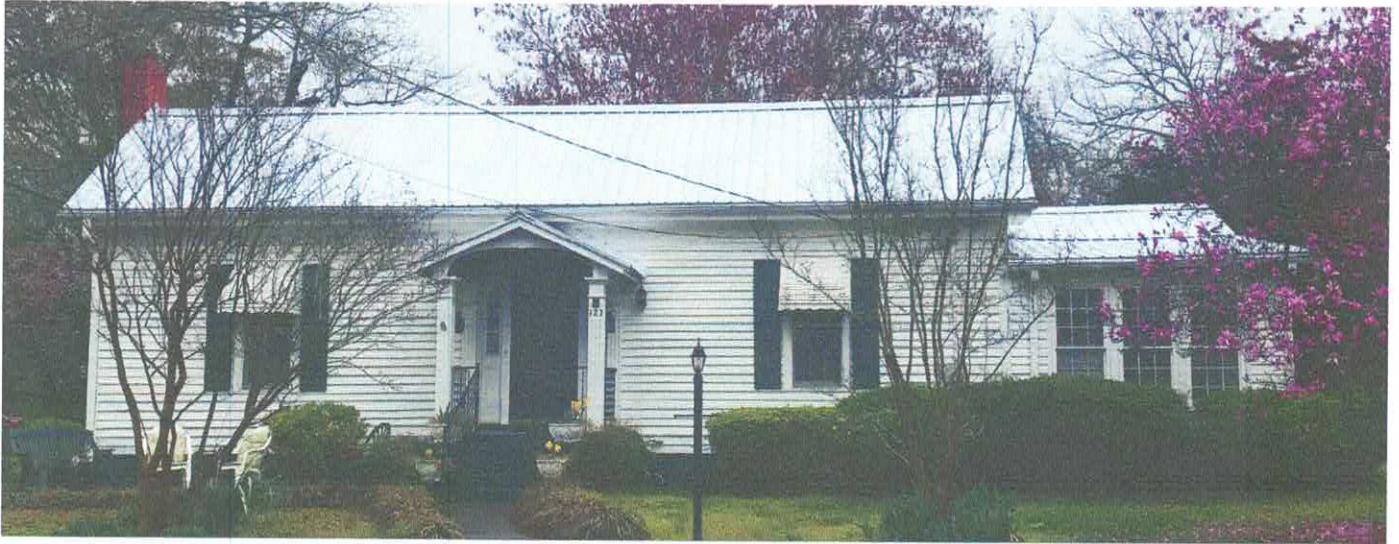
Front Western Elevation
